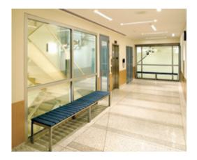
2-hour exit/stairwell enclosure providing vision and security with fire resistive glazing and framing that blocks radiant heat. The Reece School, New York City.
