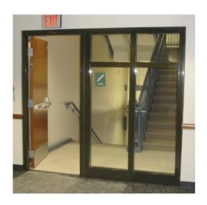
Sidelites and transoms adding light and security to a 2-hour stairwell at Ohio University.
